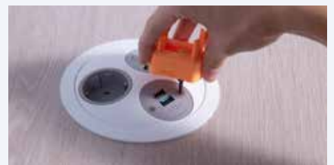
Using the TUF replacing tool and 'snake eye' bit, screw the snake eye screws back into place
